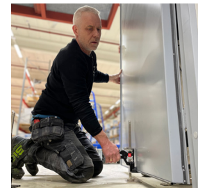
Install doors, gates, and fences. Installation de portes, clôtures et portillons.
